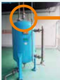
An example of the hazard and control measures: It was identified there would be a vessel overpressure hazard due to operation error. An action of lock open the vent valve was developed to control the risk.
